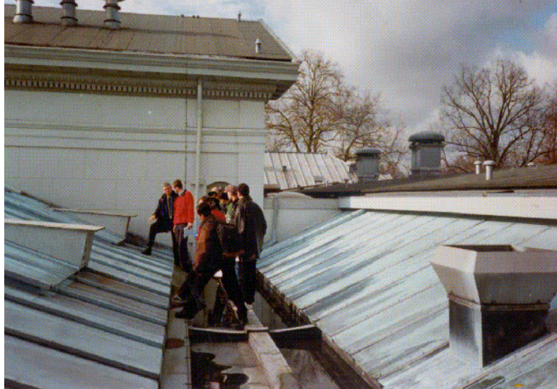
FIGURE 1. Observation of the aquarium roof.
